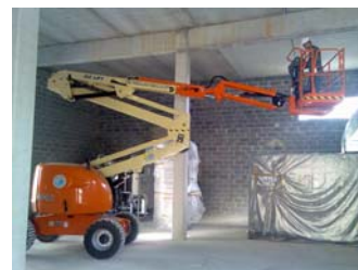
On site installation
